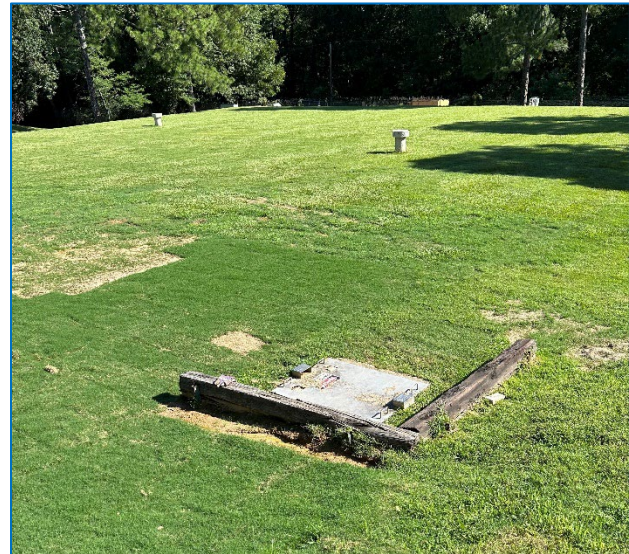
Entry Hatch – East Reservoir
